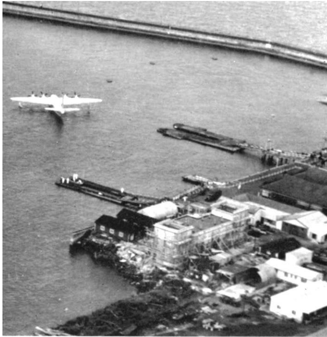
A photo from around 1950 showing the engine test building with its turrets each end.
